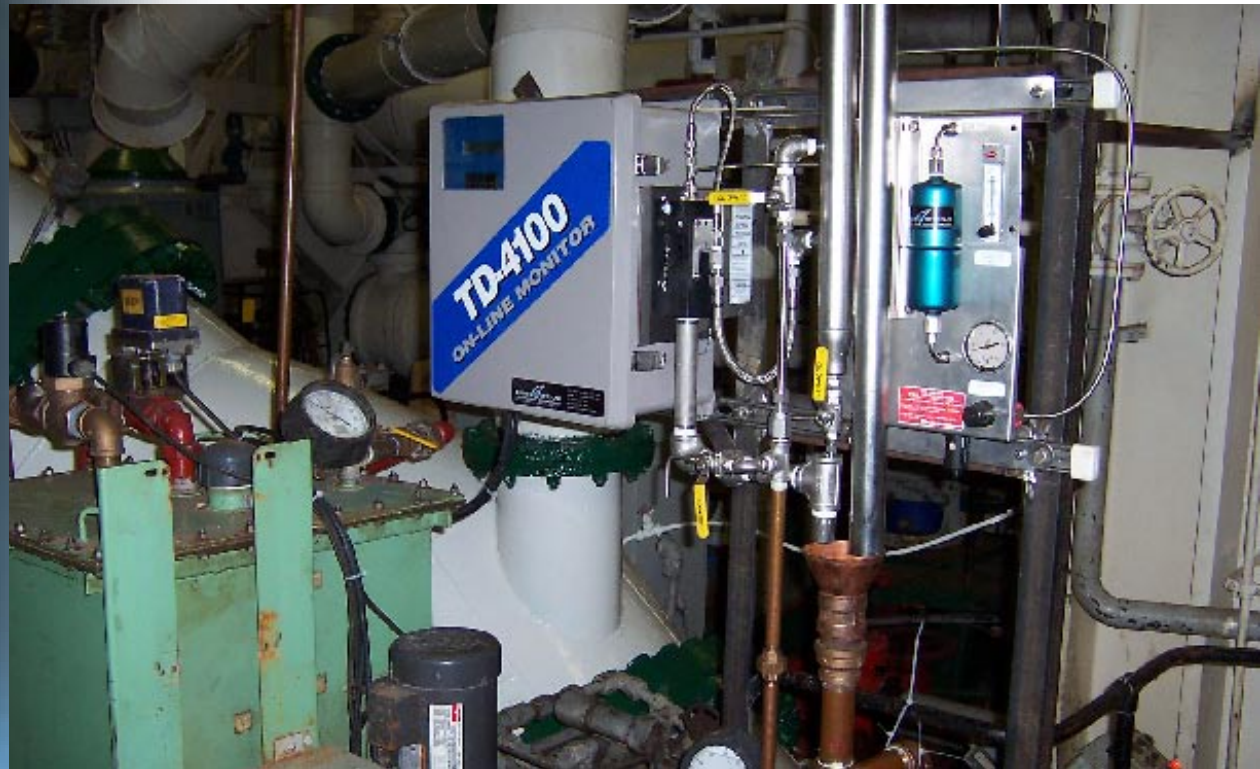
NAG installed a TD-4100 UV Fluorescence Oil Content Monitor on the OWS of SS Stephen W Pless
